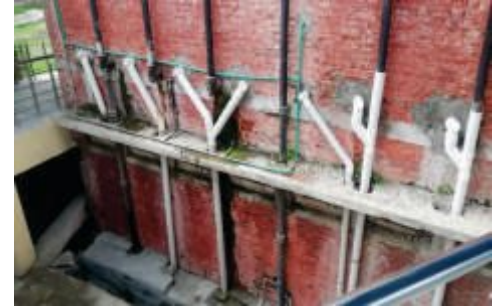
New pipes for sewerage
